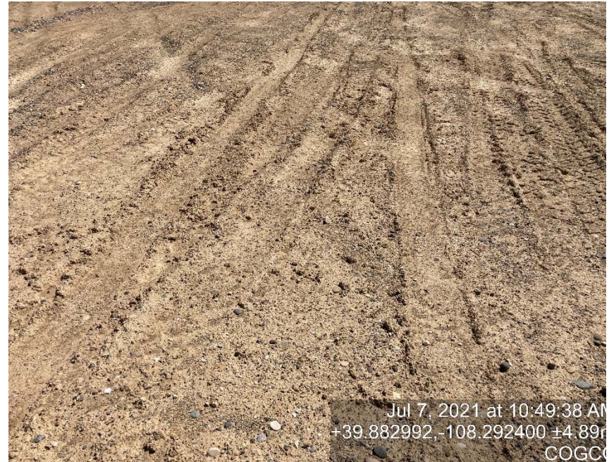
Lack of stabilization/compaction
