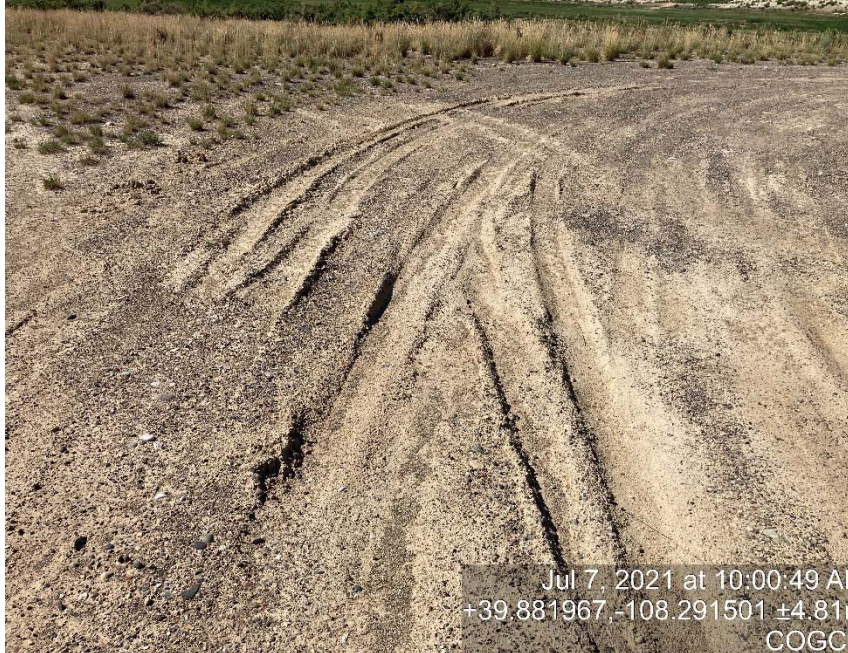
Lack of stabilization/compaction
