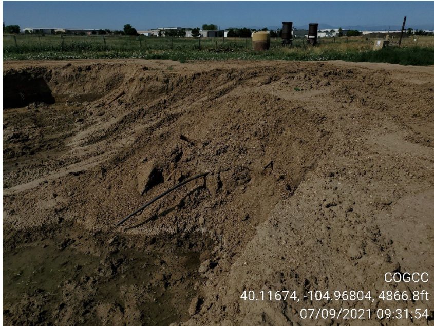
Photo 3 Eastern excavation, looking at flowlines exposed in western excavation wall
