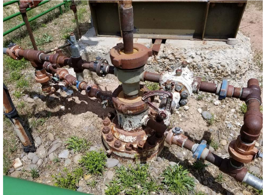
Photo 2. No bradenhead access apparent.
