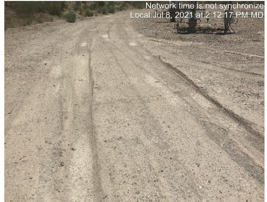
Photo #4366 Location lacks stabilization.
