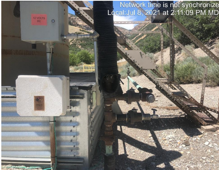
Photo #4365 Heating insulation opened ended and not capped.
