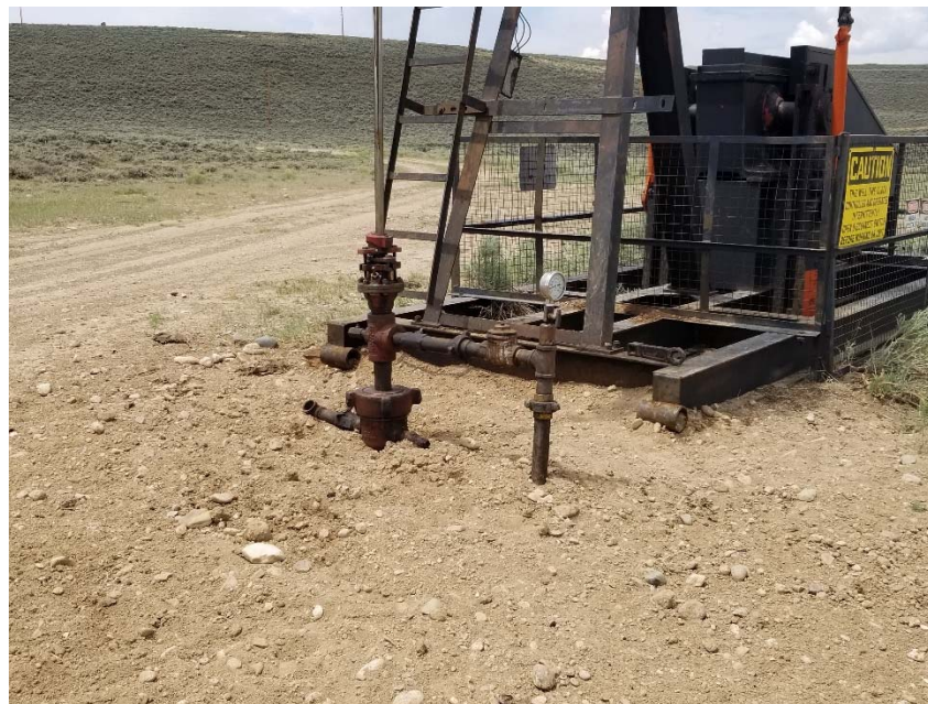
Photo 2. No bradenhead access apparent.
