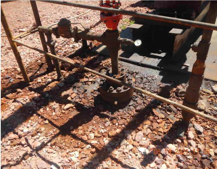
Photo #2 contaminated soil at wellhead.
