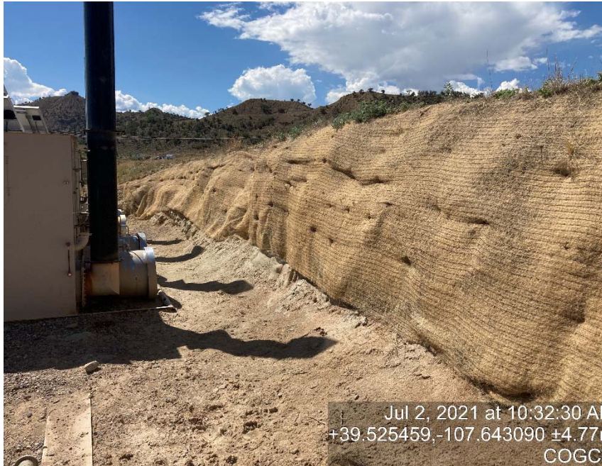
Location/matting on cut slope behind separators
