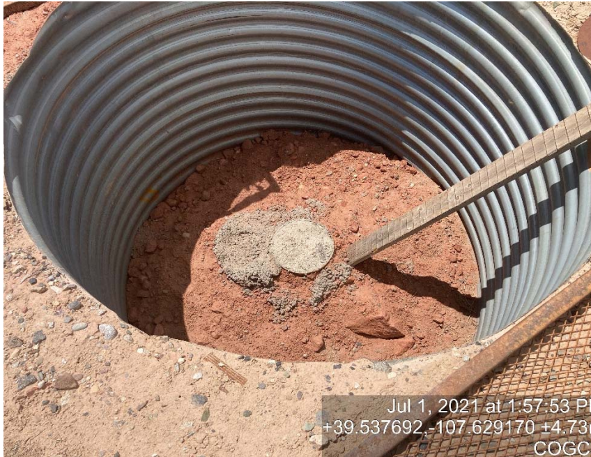
Open holes for wild life/livestock to fall into (fencing not adequate)
