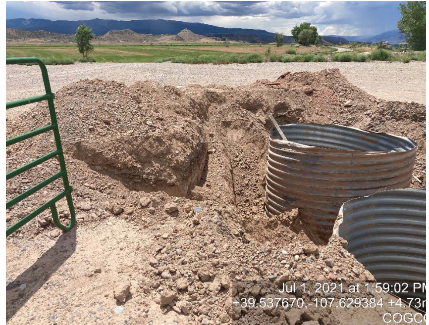
Open holes for wild life/livestock to fall into (fencing not adequate)
