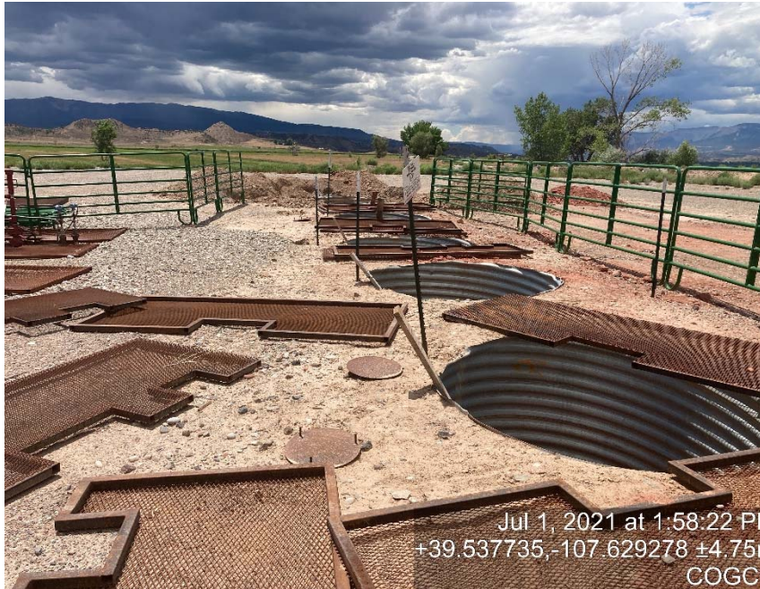
Open holes for wild life/livestock to fall into (fencing not adequate) and debris
