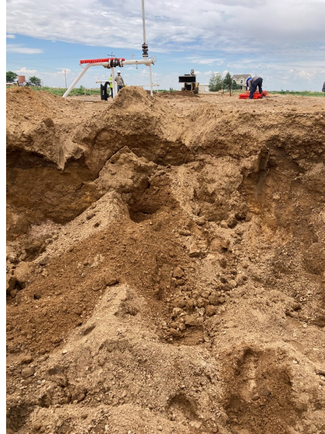
Looking west-southwest at eastern separator/dumpline connection area No petroleum hydrocarbon odor or staining observed in soil
