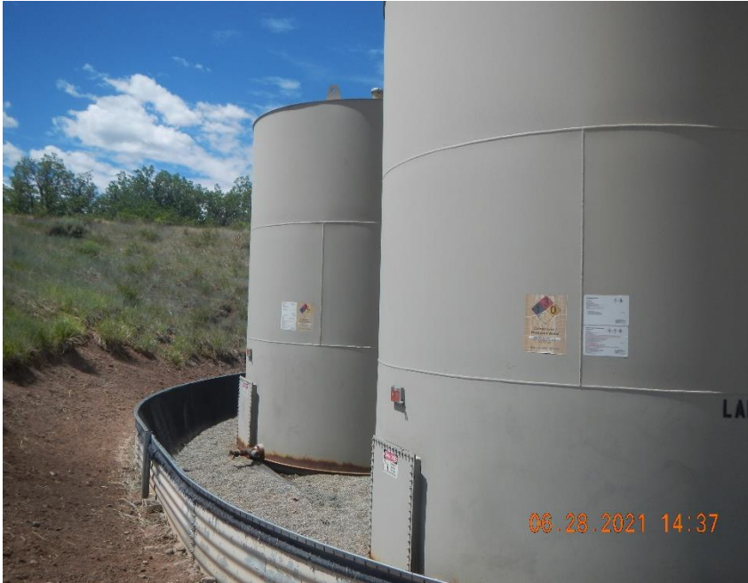
Tank labels are weathered and illegible from a distance. (100')
