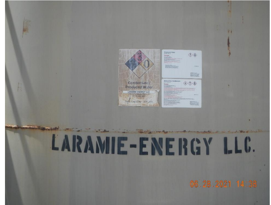
Tank labels are weathered and illegible from a distance. (100')
