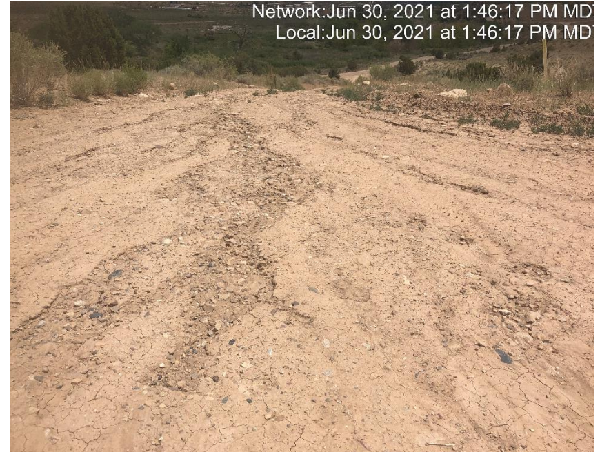
Photo #4249 No form of tracking BMP at entrance to location.
