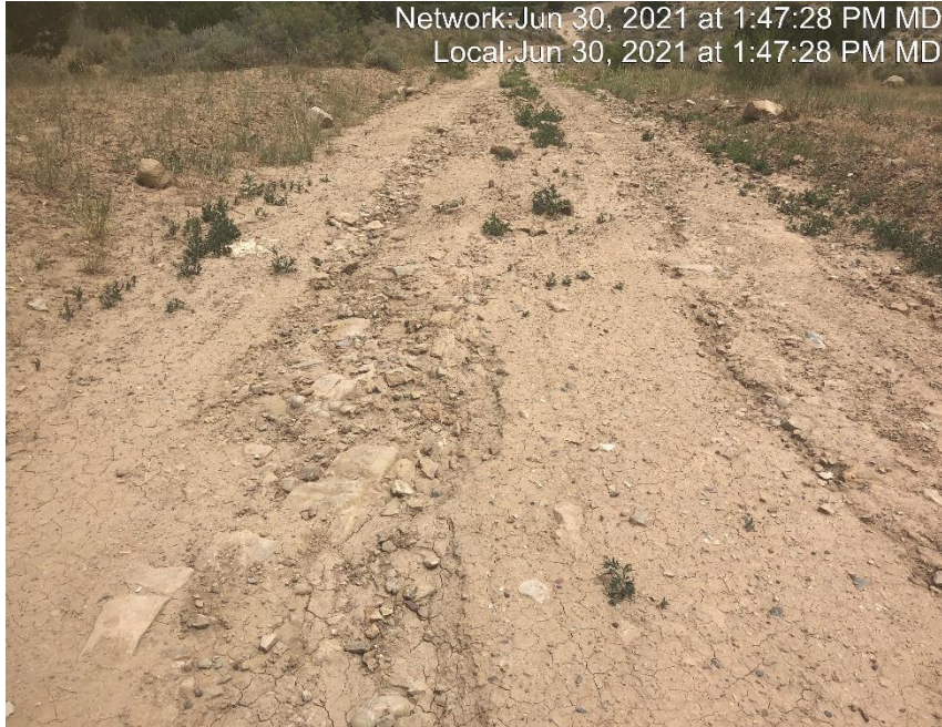
Photo #4250 Rill erosion occurring in center of access road.
