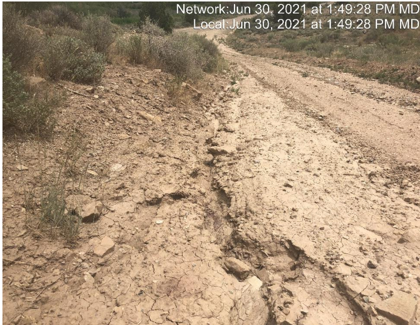
Photo #4253 No velocity checks located in access road ditches.
