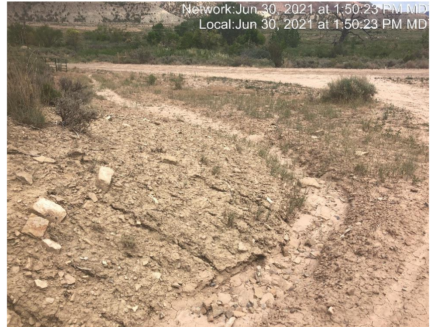
Photo #4254 Gully erosion occurring at entrance to access road.
