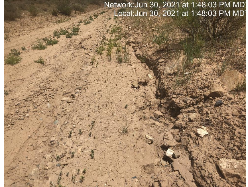
Photo #4252 Rill erosion occurring in access road ditches.
