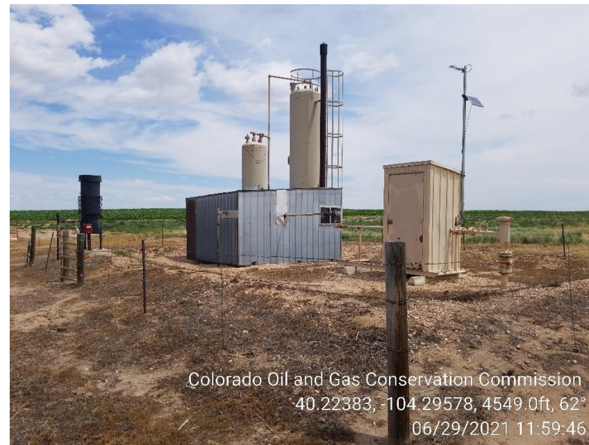
Photo 2 – Heater Treater, Gas Meter and ECD
