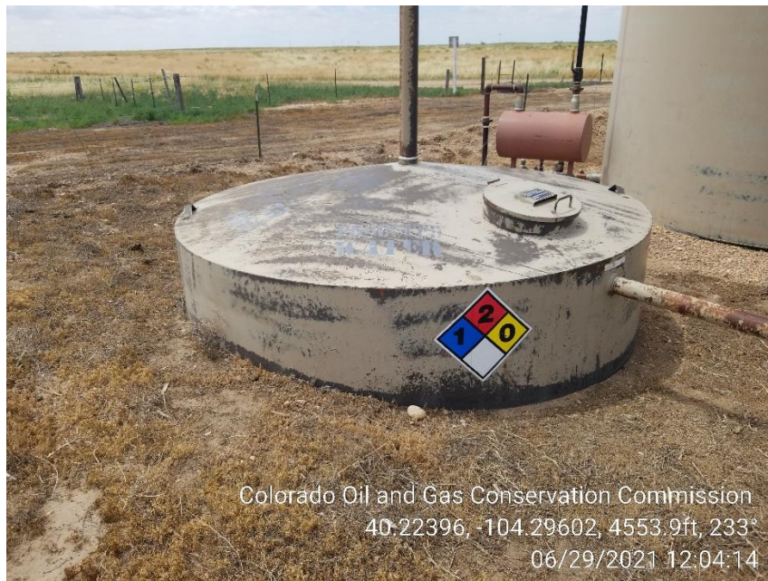
Photo 5 – Produced Water Tank
