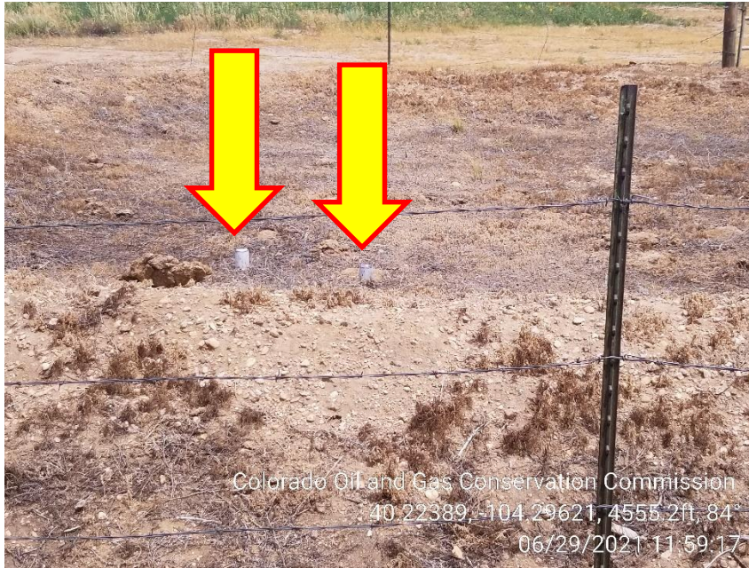
Photo 9 – Unmarked Risers
