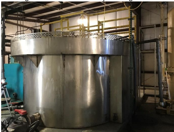
Former DAF Used as Backwash Storage Tank
