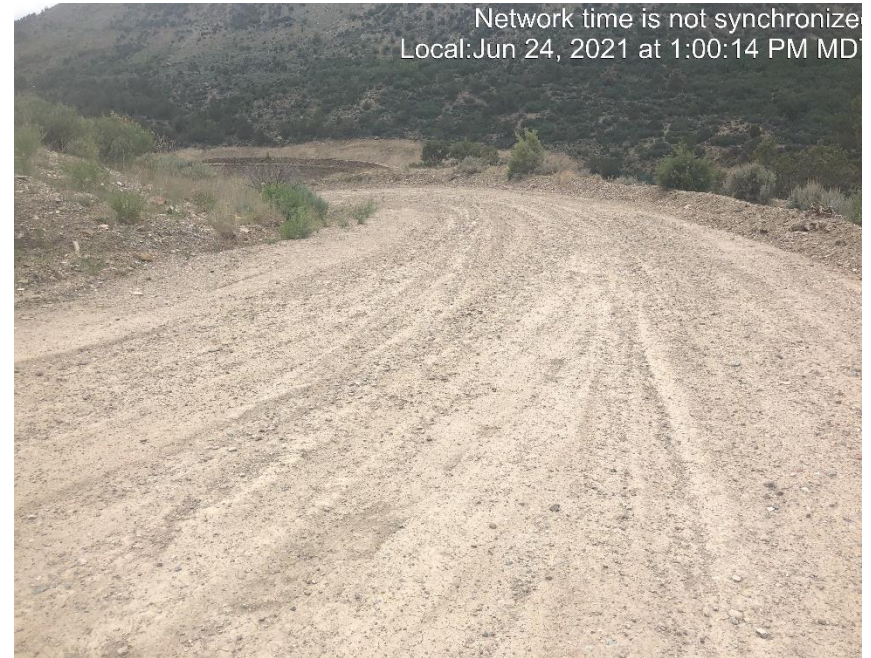
Photo #4170 No form of tracking control located at the entrance to location
