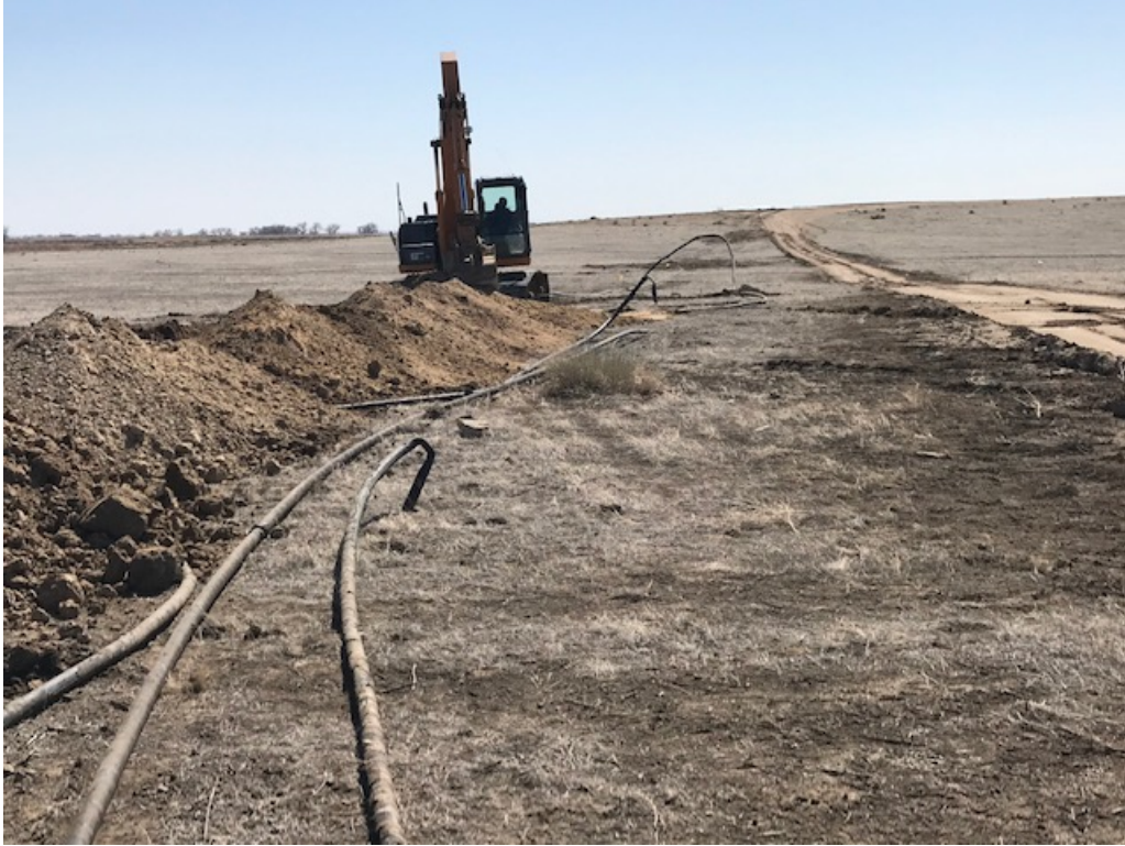
#9 - Looking Southwest at the Open Trench used for Pipe Removal
