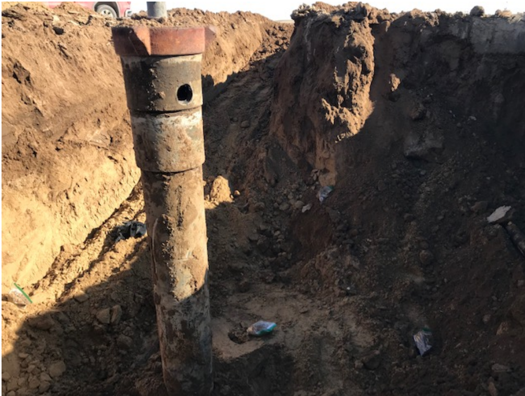
#2 - Wellhead Prior to Cut & Cap. Soil Samples have been collected.
