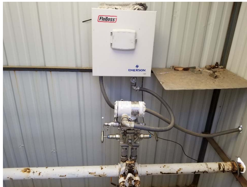
Photo 4. No meter calibration displayed.
