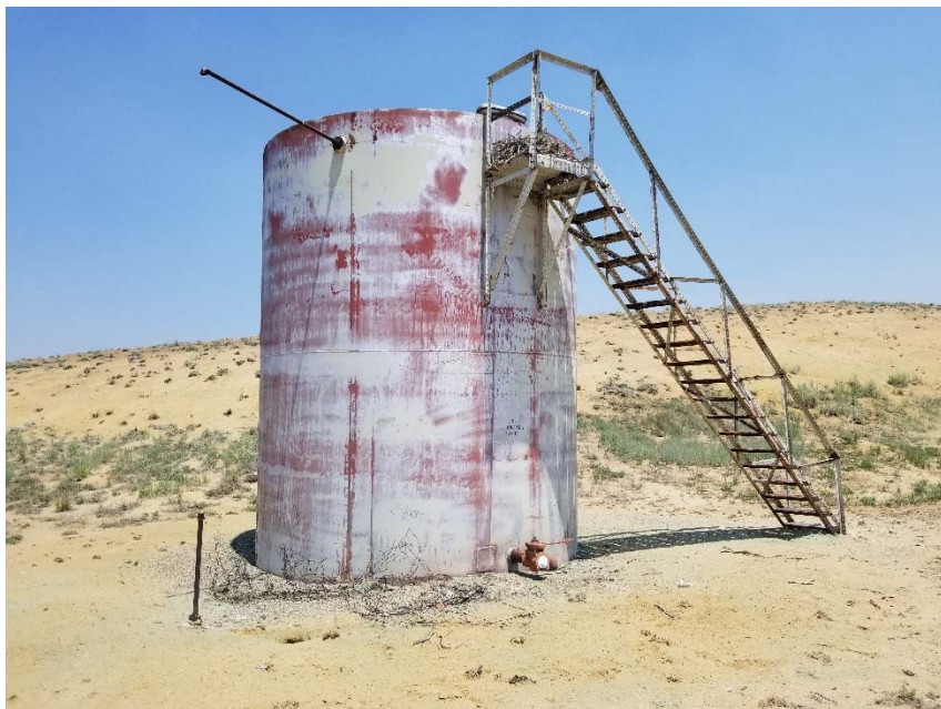
Photo 3. No tank label. No berm.
