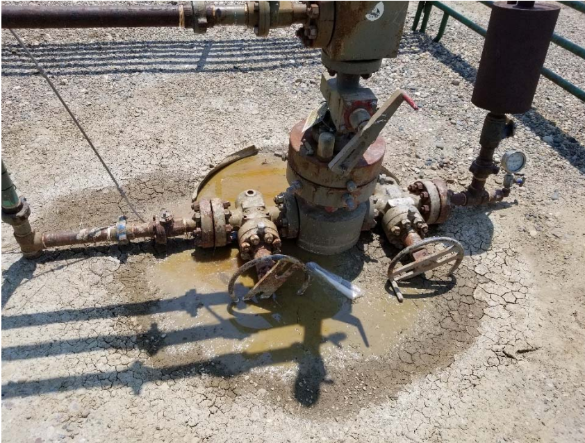
Photo 2. Standing water in cellar. Possible leak.
