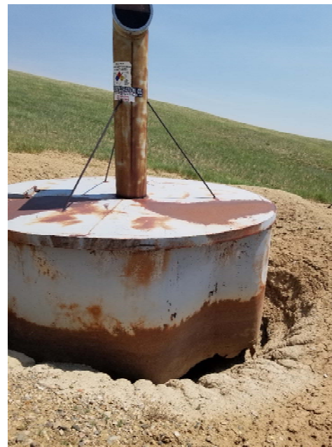
Photo 2. Hole in produced water tank.
