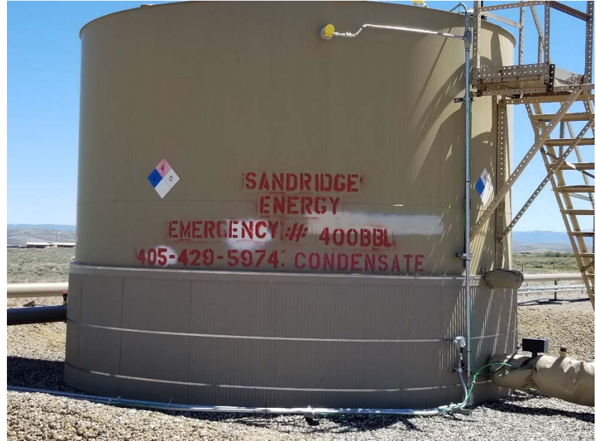
Photo 5. Tank label inaccurate.
