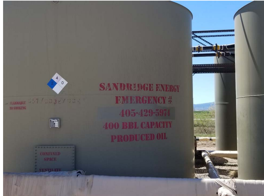
Photo 3. Tank labels incomplete.
