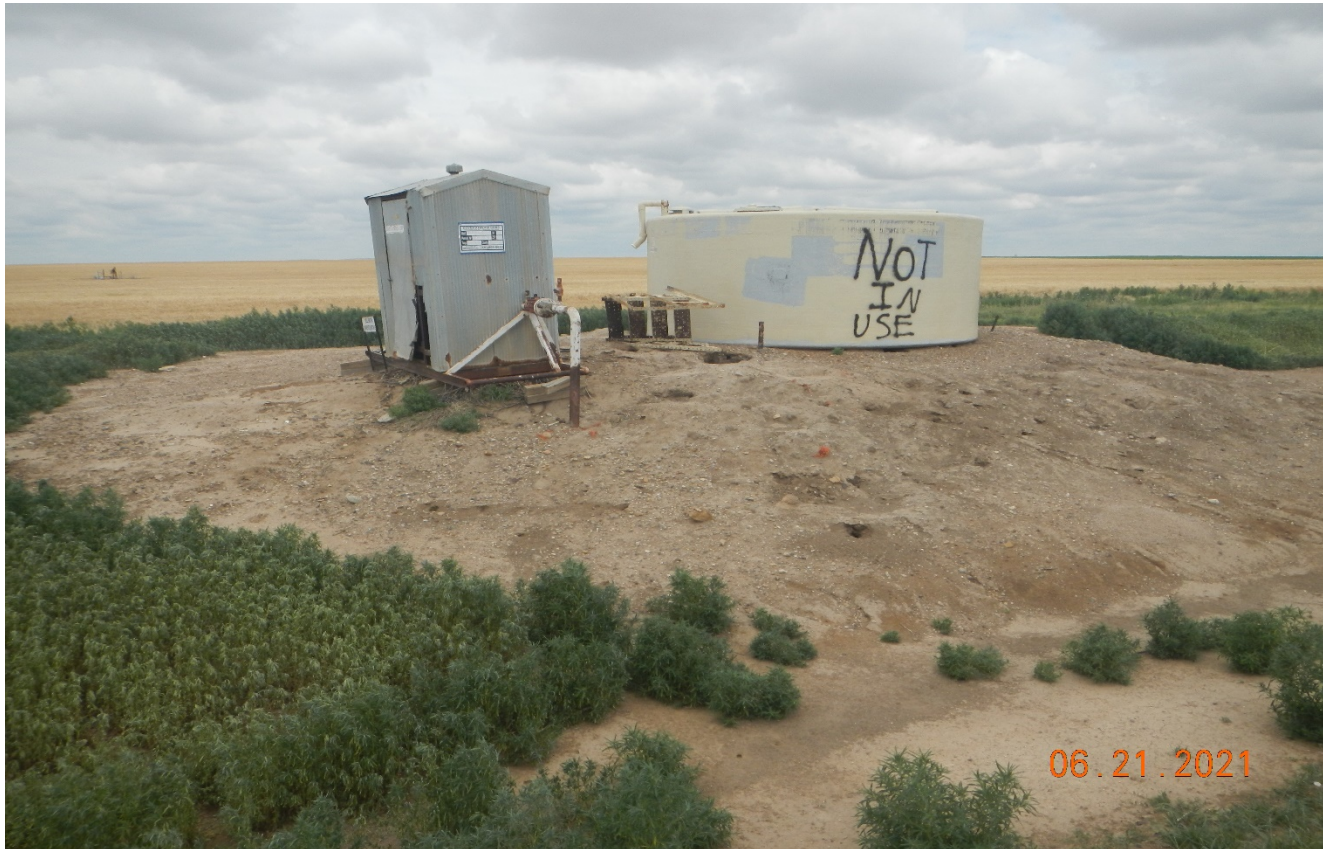
Photo 1. Facing west toward the PW tank and meter shed located adjacent to CR-49 and 575' east of the well. No operator sign is visible from the county road but a sign was observed on backside of tank. Meter shed still appears to be unstable and there is no berm around the tank. Corrective actions were not completed.
