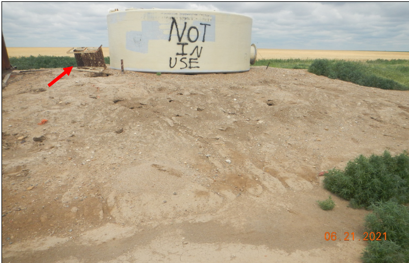
Photo 4. Corrective actions of the previous inspection were not performed. There is no berm around the 200 bbls tank. There is unused equipment at the location (red arrow). There is erosion occurring around the tank area.
