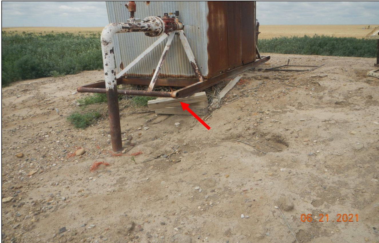
Photo 3. The meter shed is not maintained and remains unstable. Erosion has occurred underneath the meter shed which is a safety concern. Wood blocks are ready to fall over shown at red arrow.
