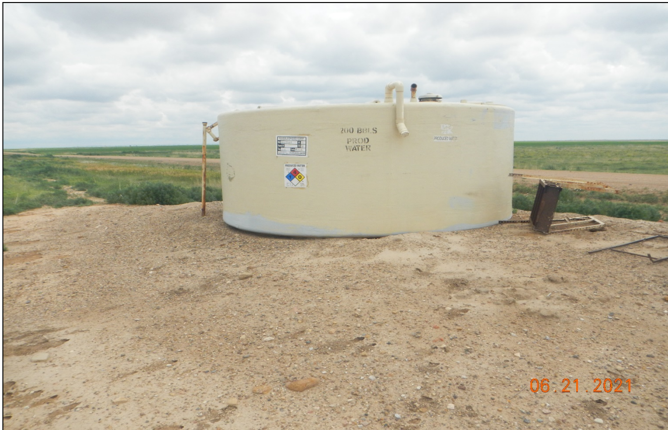
Photo 5. The tank sign and NFPA label are installed on backside of the tank which is not readily visible from the front side along the county road.
