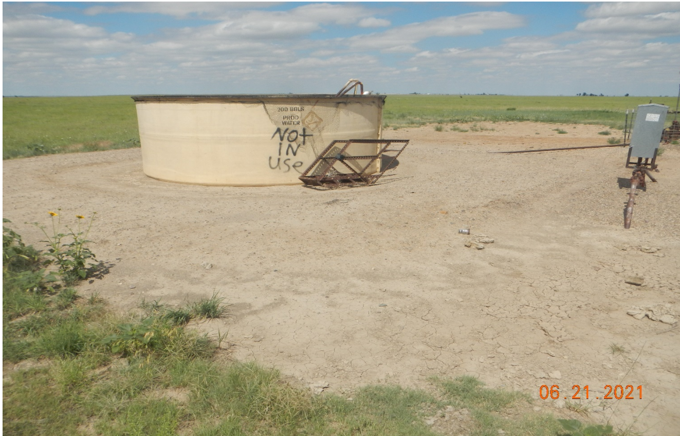
Photo 2. The tank is marked as not in use and labeled Produced Water. Next photo shows oily fluids inside the tank which apparently the tank is in use. Secondary containment is inadequate to contain 150% of the volume of the tank.
