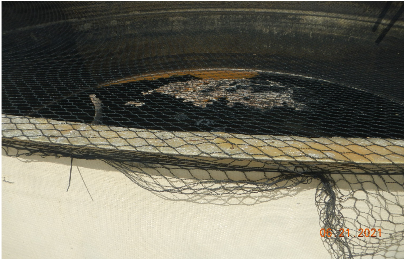
Photo 3. View of oil fluids inside the tank. Tank is labeled Produced Water which is not accurately labeled.
