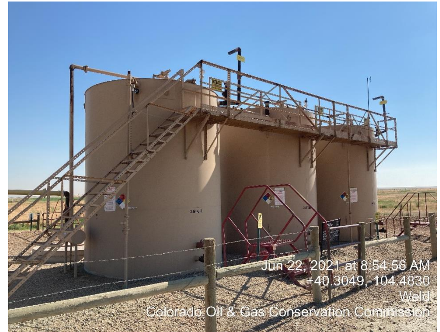
Photo #3 Tank Battery
