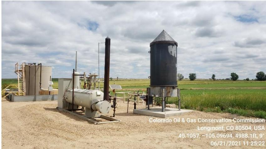
**Photo 7 ECD and Horizontal Heated Separator**
