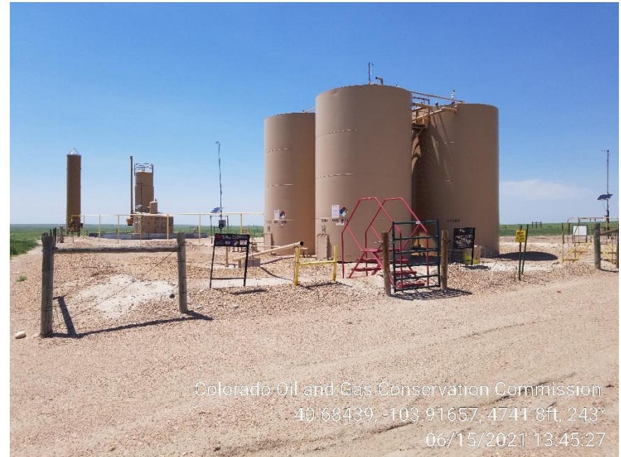
Photo 4 – Tank Battery
