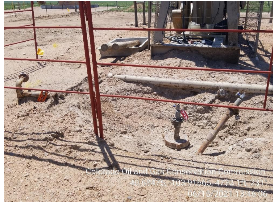
Photo 2 – Well Plugged and Abandoned
