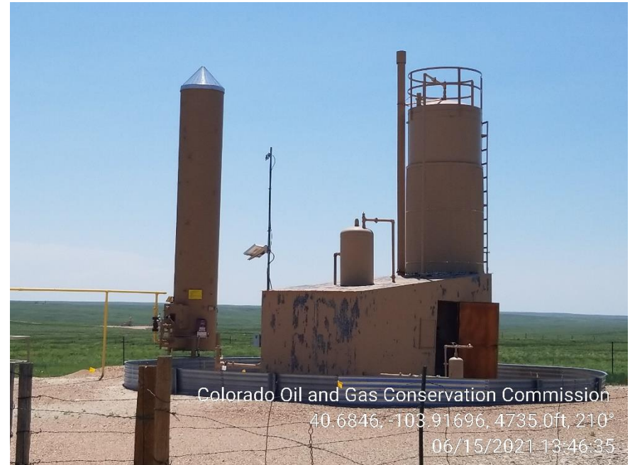
Photo 6 – Heater Treater and ECD
