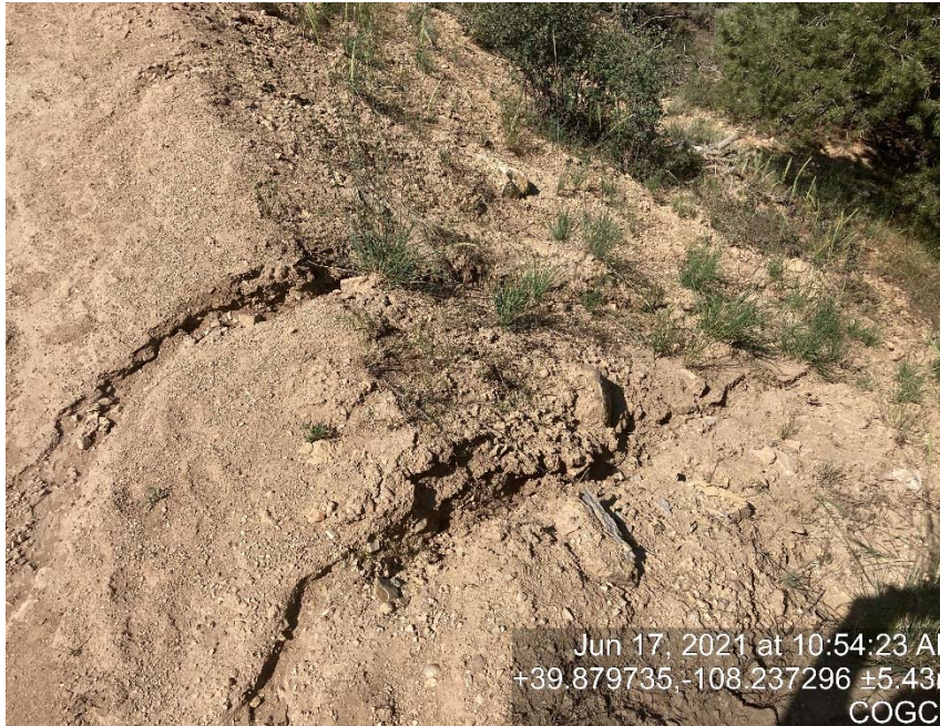
Erosion is occurring on access road
