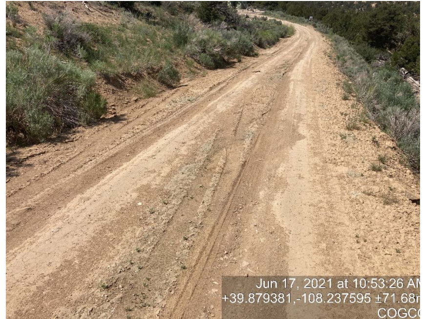
Erosion is occurring on access road and not stabilized/compacted
