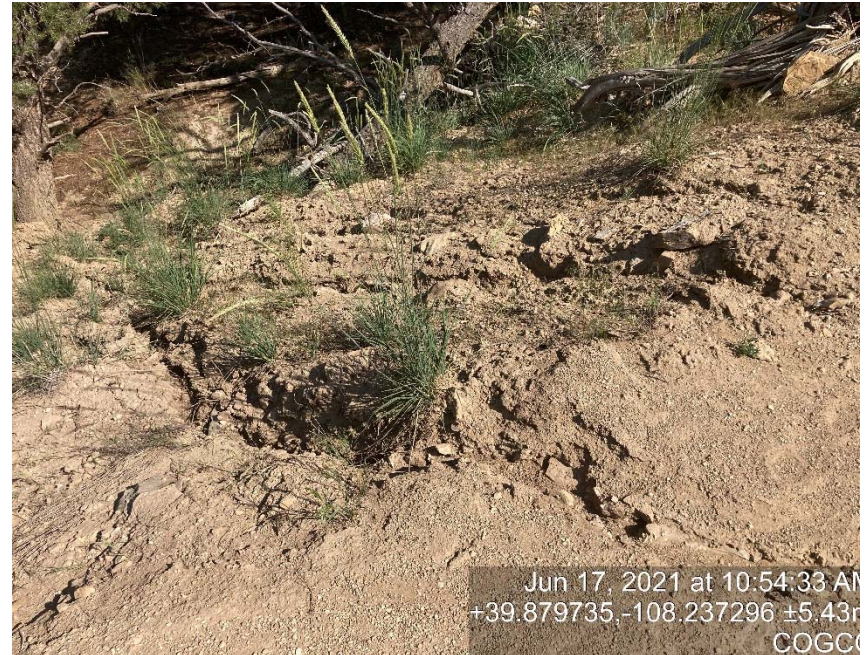
Erosion is occurring on access road
