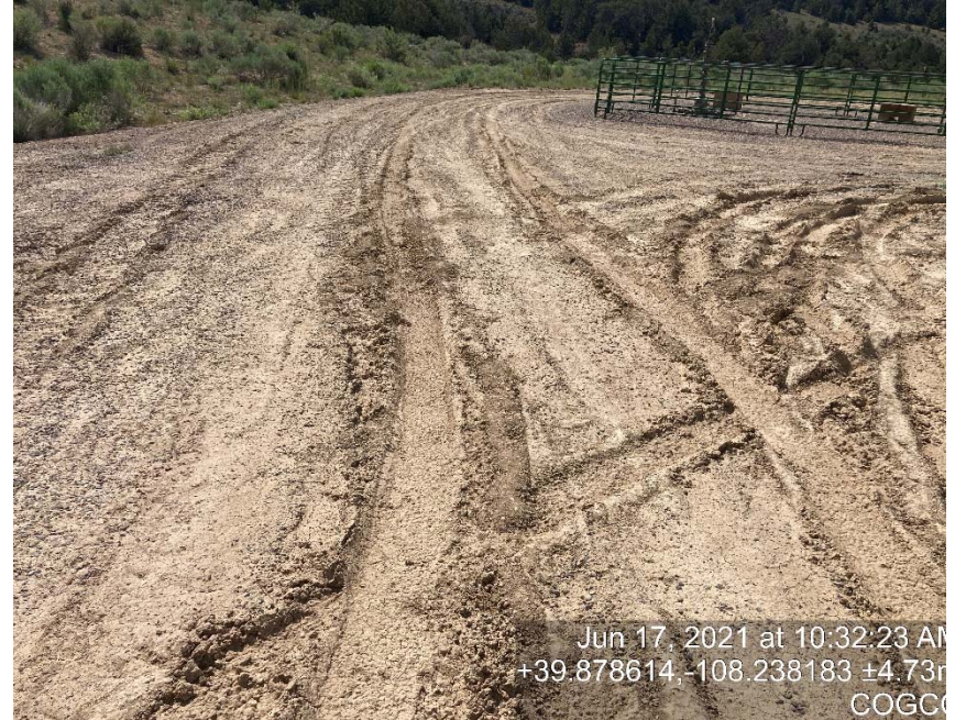
Lack of stabilization/compacted
