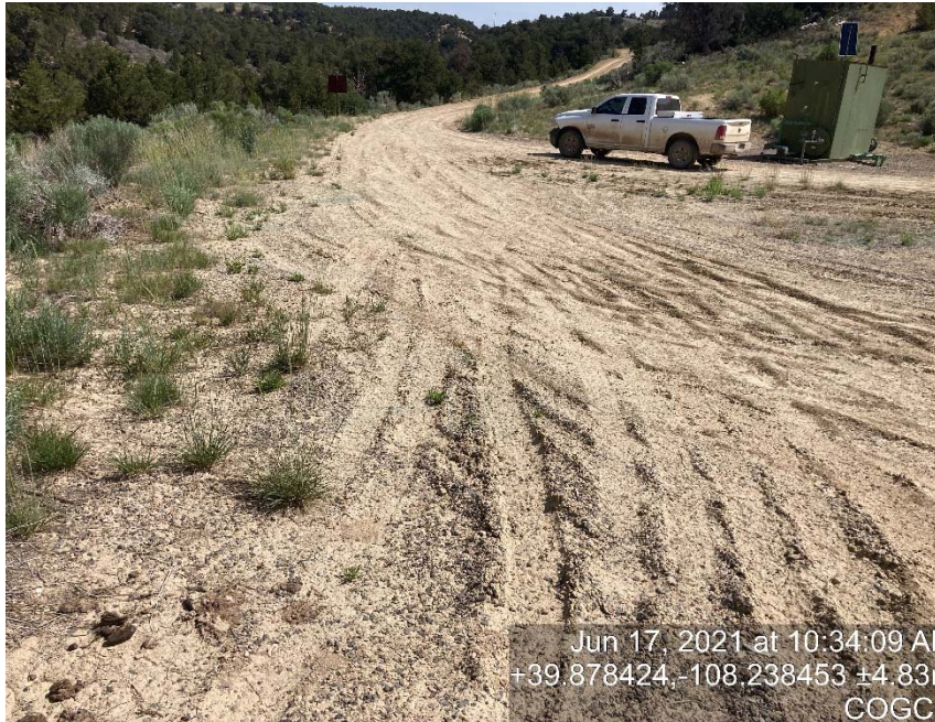
Lack of stabilization/compacted
