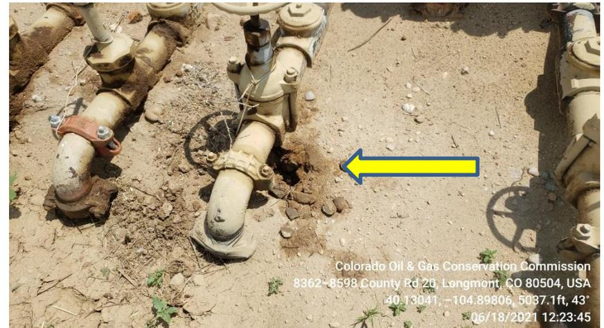
**Photo 17 Stained soil by flow line manifold**
