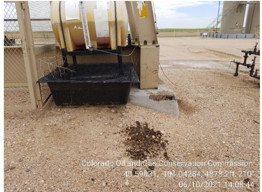
Photo 8 – Stained Soil at Wellhead
