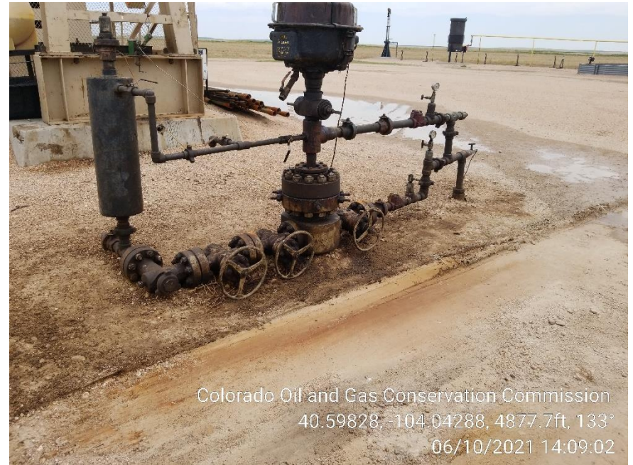
Photo 10 – Stained Soil at Wellhead
