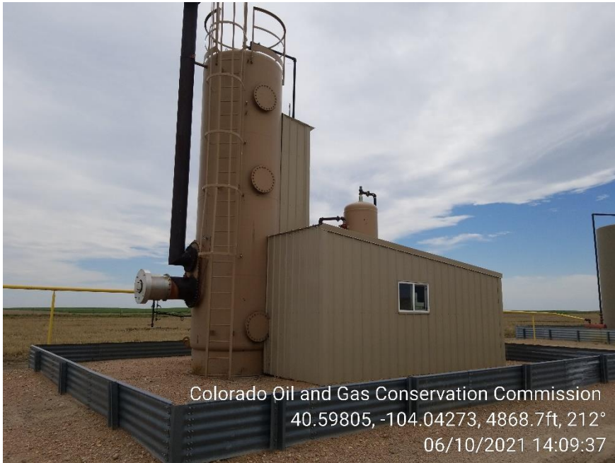
Photo 5 – Heater Treater
