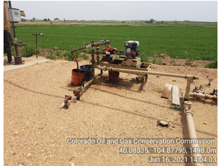
Photo 2 Recirc pump. Stained soil and mechanical issues.
