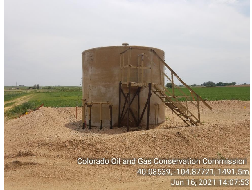
Photo 6 Produced water tank not placards or labels.
