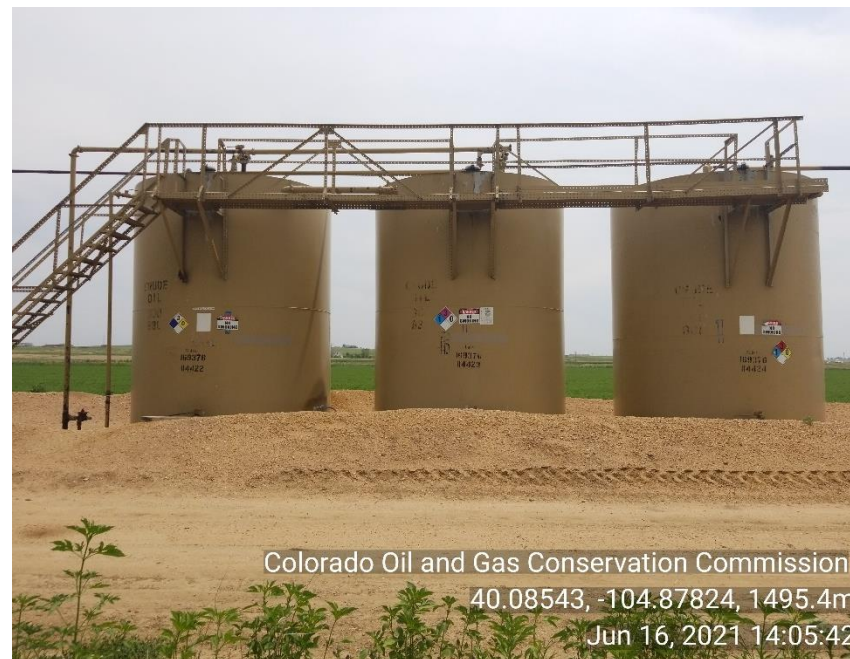
Photo 4 Labels and placards faded not readable.
