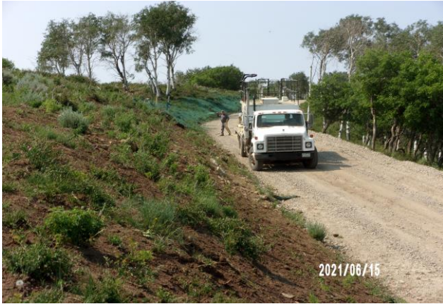
Applying Hydrmulch on the CC 697-03-07 Access Road
