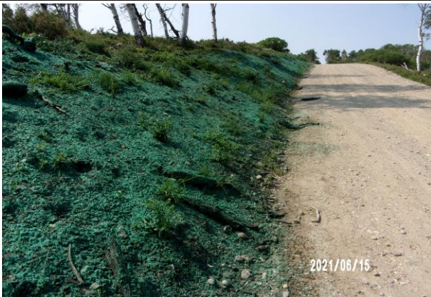
Hydromulch Application on the CC 697-03-07 Access Road
