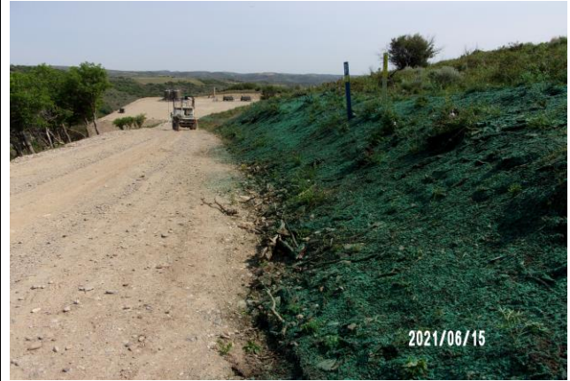
Applying Hydrmulch on the CC 697-03-07 Access Road
