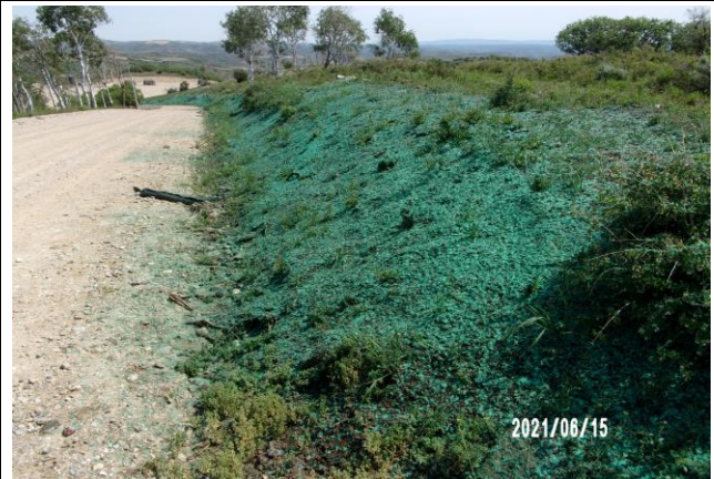
Hydromulch Application on the CC 697-03-07 Access Road
