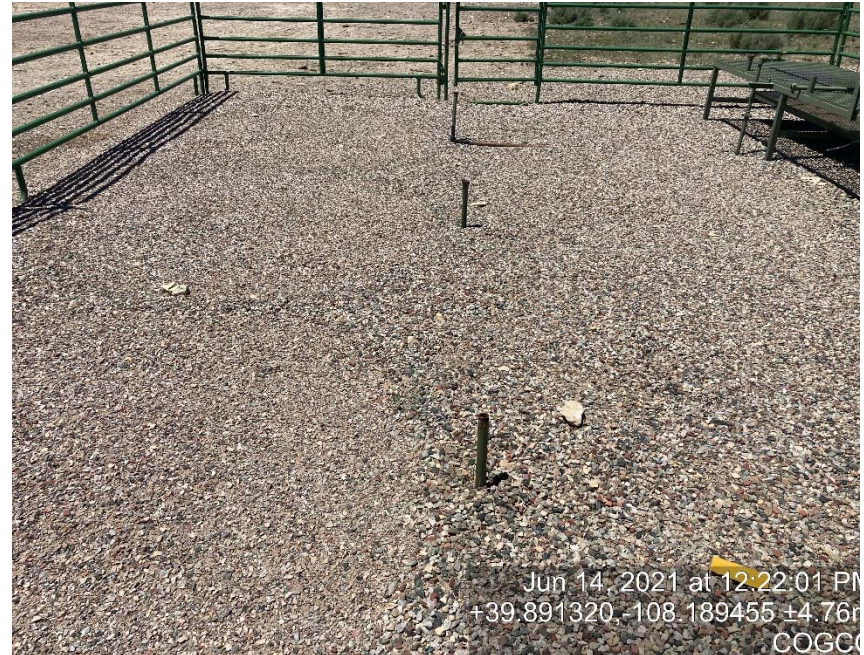
Piping from chemical tanks is disconnected
