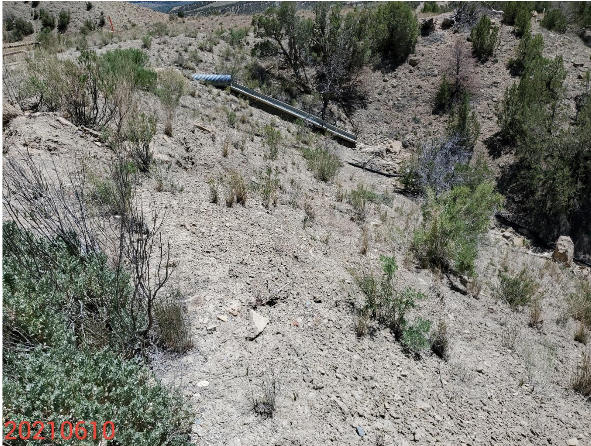
Photo 1: Photo taken from the slopes on the west end of the Location, facing south. Photo shows control measures to protect/stabilize slopes remain missing or insufficient.
