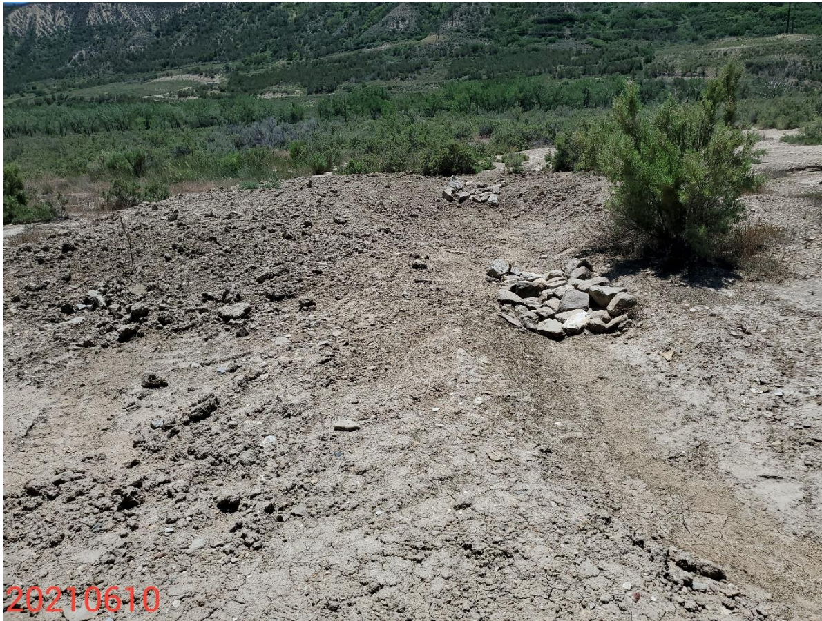
Photo 3: Photo taken from the south end of the Location, facing south. Photo shows Operator has implemented a sediment trap; inlet/outlet of trap observed to be constructed with a geotextile lining and rock armoring.
