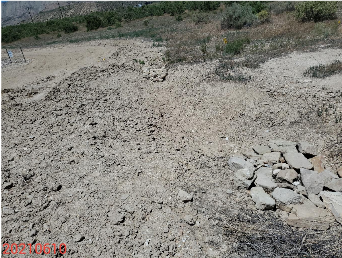
Photo 4: Photo taken from the east end of the Location, facing north. Photo shows Operator has implemented a sediment trap; inlet/outlet of trap observed to be constructed with a geotextile lining and rock armoring.
