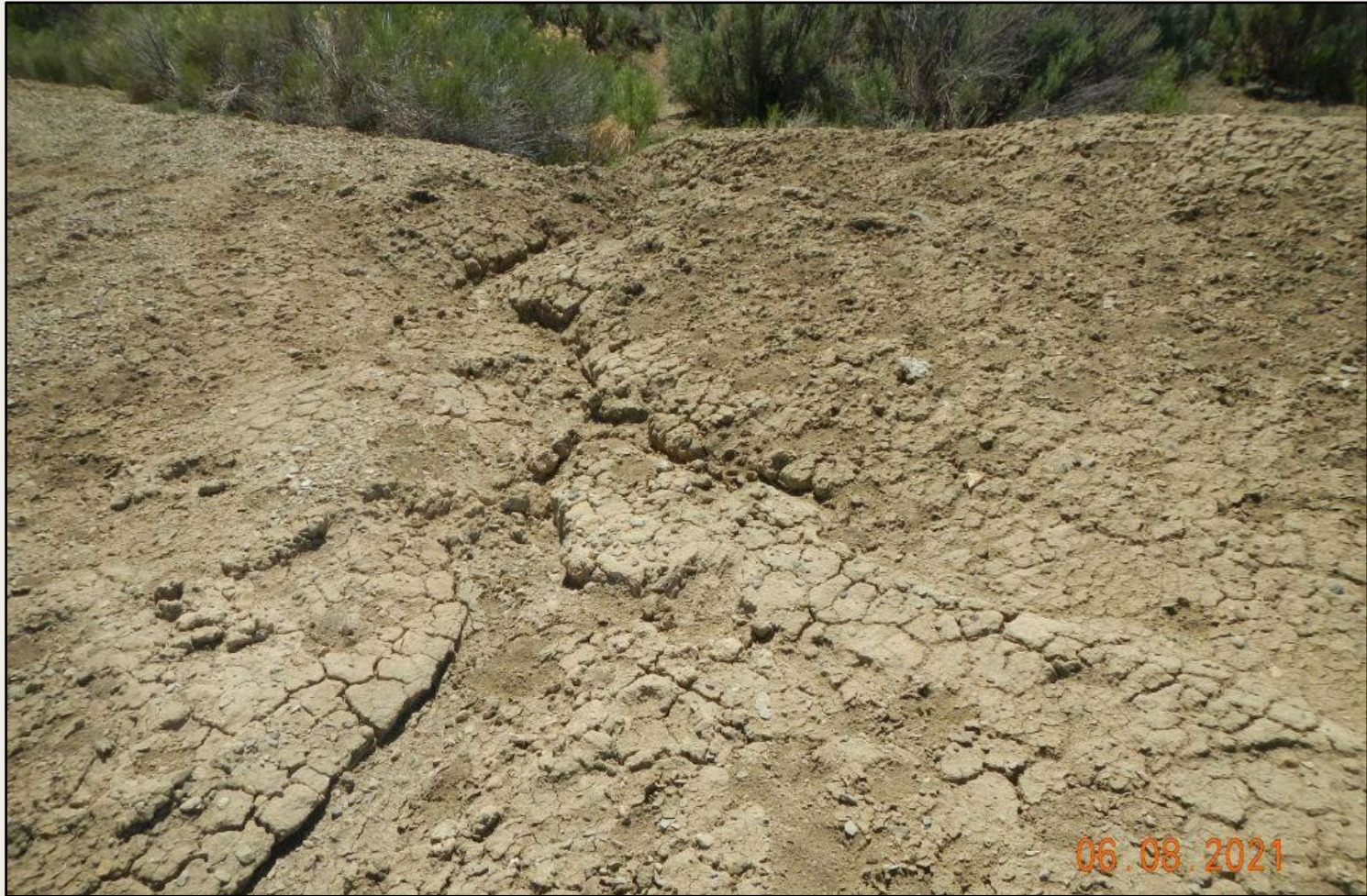
Photo 3. View of erosional channel forming where concentrated stormwater runs off of the northwestern edge of the well pad. Channel is approximately 6-8 inches wide and deep.
