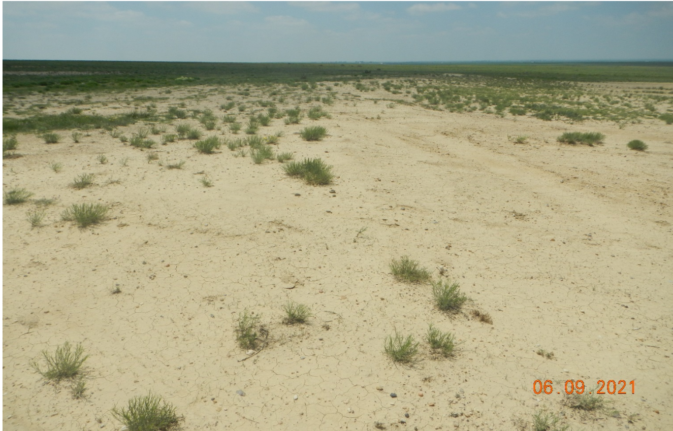
Photo 3. Facing southwest at the location. The fill slope has not been recontoured. There is no vegetation growth along this area.
