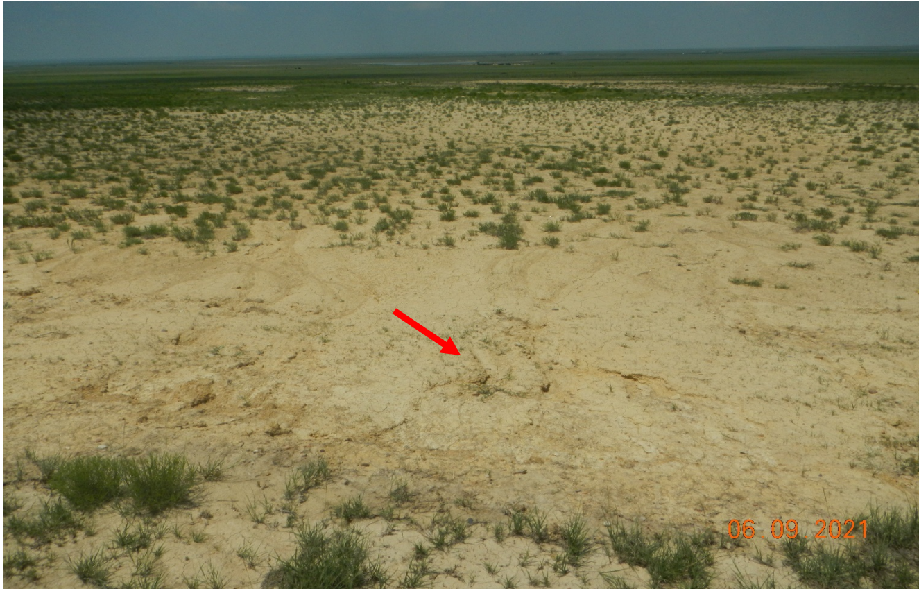
Photo 8. Facing north at the cut slope. Soil has been replaced along the cut slope. There is some signs of erosion and soils are not stabilized (Red arrow).
