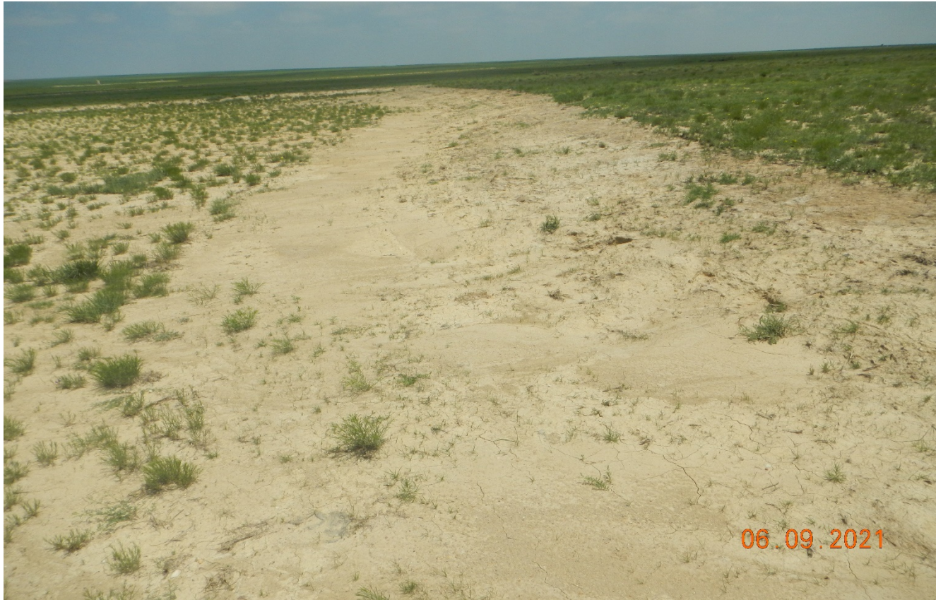
Photo 7. Facing northeast along the cut slope. Soil has been replaced along the cut slope. There are some signs of erosion and soils are not stabilized.
