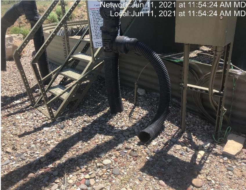
Photo #4067 Multiple flow line heating insulation open ended and not capped.
