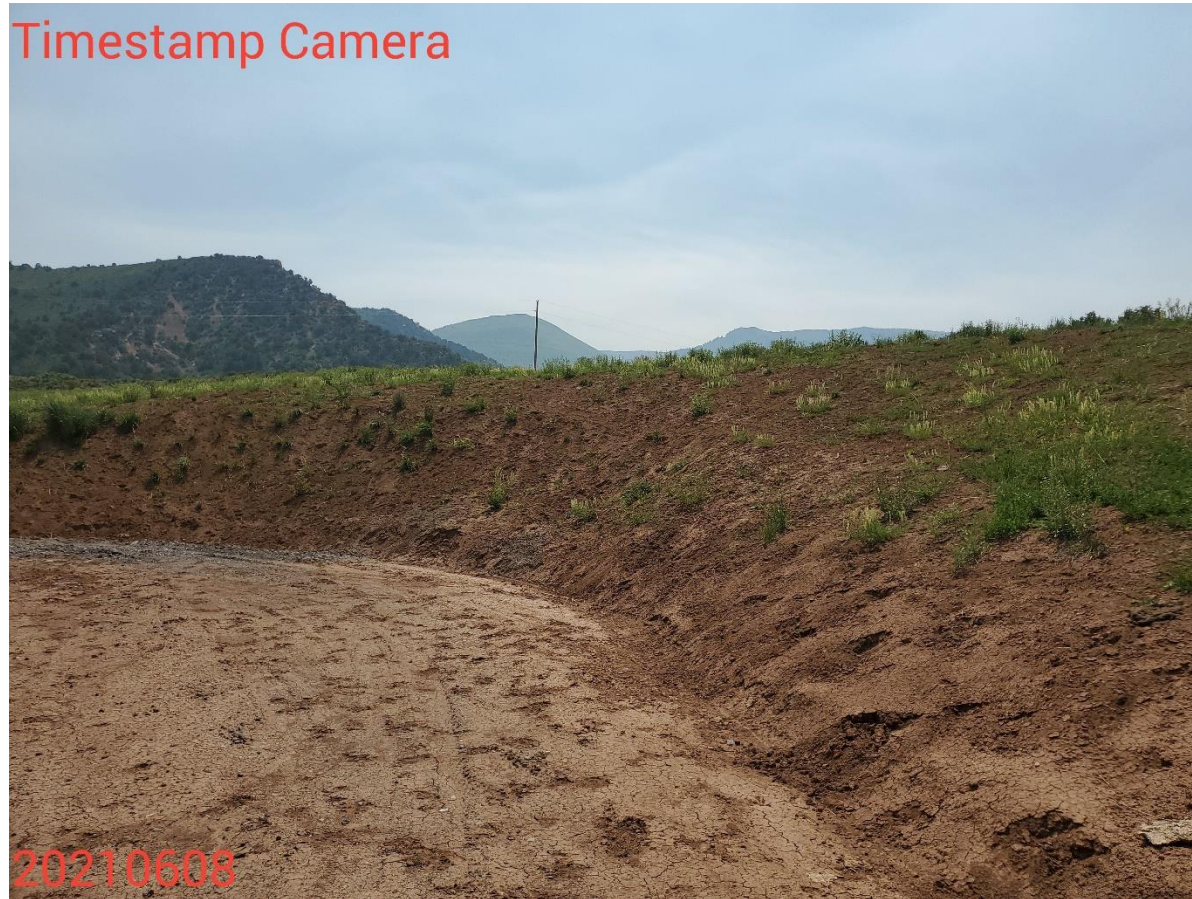
Photo 1: Photo taken from the cut slopes on the south end of the Location, facing east. Southern areas of the Location are not progressing towards 1003 standards. Areas require additional revegetation activities and control measures to stabilize soils until longer term stabilization is achieved.
