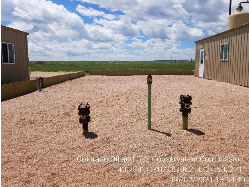
Photo 7 – Unmarked Risers South of Heater Treaters
