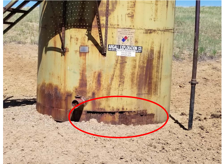
Photo 4. Close up of corrosion in tank from photo 3.
