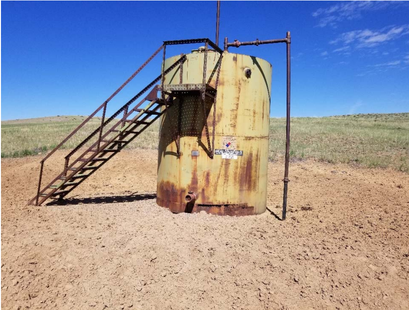
Photo 3. Produced water tank with corrosion. Tank does not appear to be in use. Tank must be removed if not in use.
