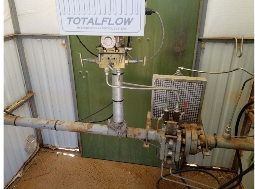
Photo 4. No calibration in gas meter run.
