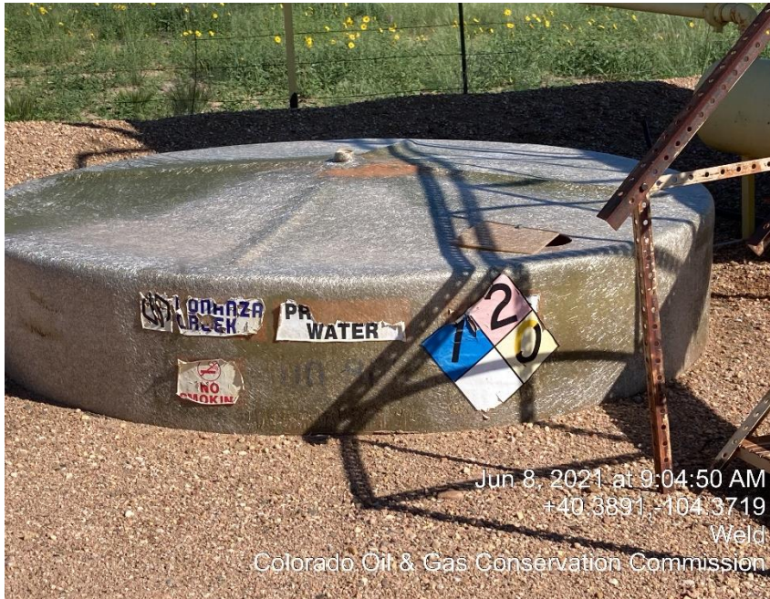
Photo #4 Weathered labels & Missing capacity label
