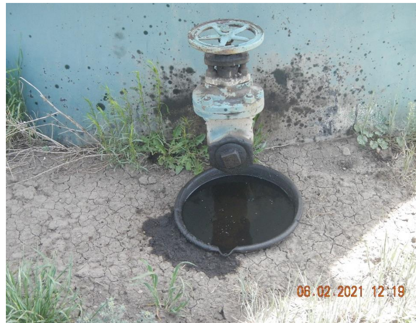
Drip pan is overflowing.
