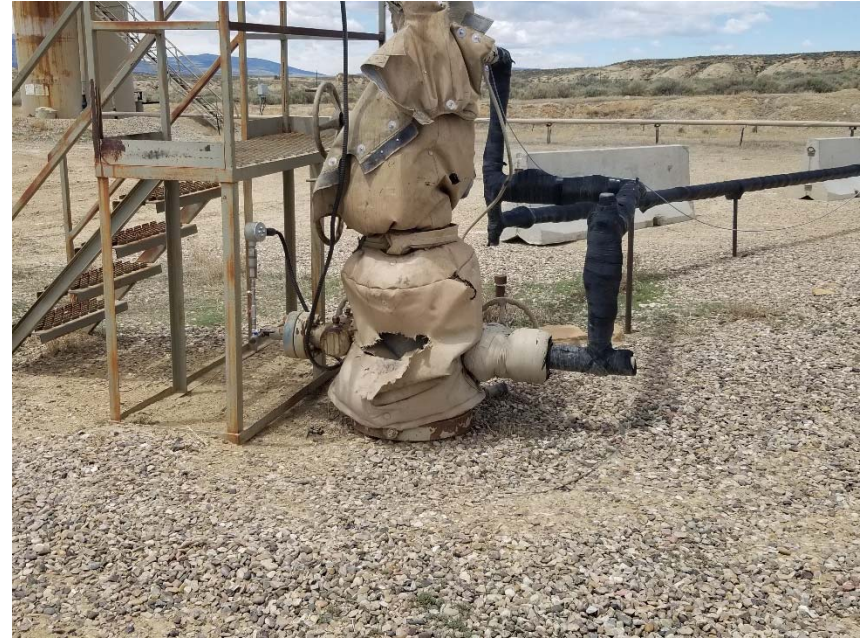
Photo 2. No bradenhead access apparent.
