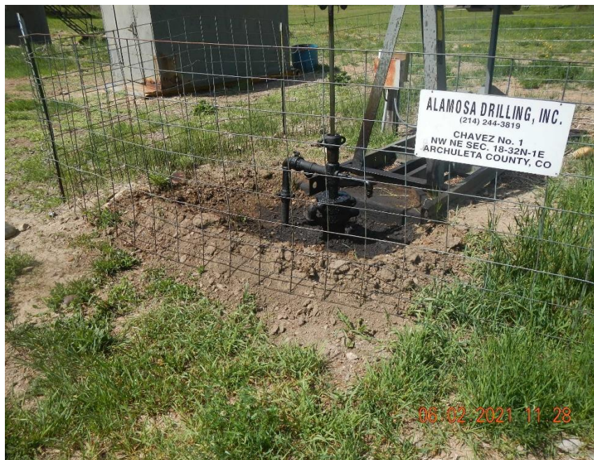
Chavez #1 well head and surroundings are stained and wet.
