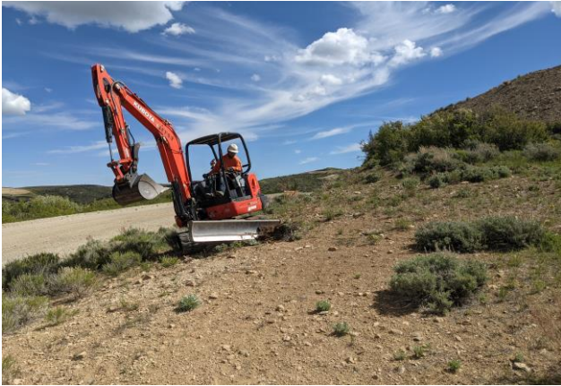
Installing Trench to Key-In Wattle Installations
