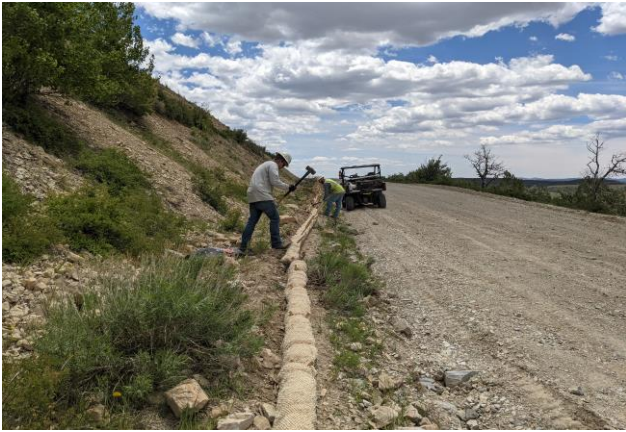
Installing Wattle along Access Road
