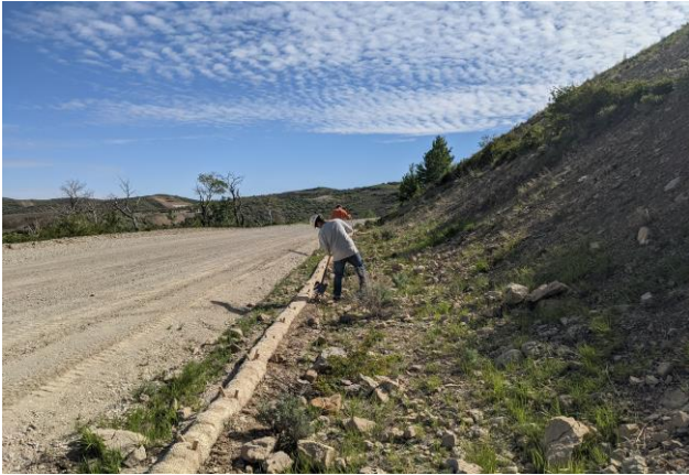
Backfilling Wattle Installed Yesterday on CC 608-43-31 Pad
