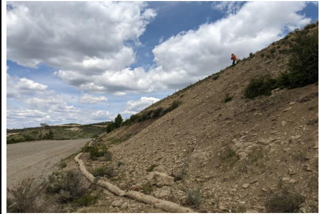
Excelsior Wattle Installed below Fill Slope
