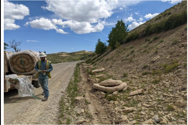
Wattle Trench Installed below Fill Slope
