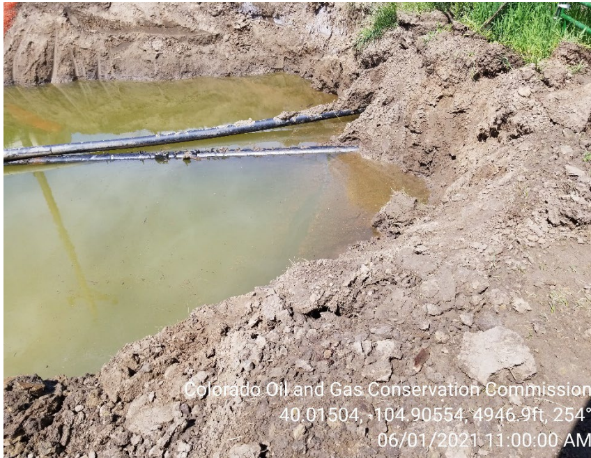
Photo 3 – Open excavation. Hydrocarbon sheen observed on groundwater.
