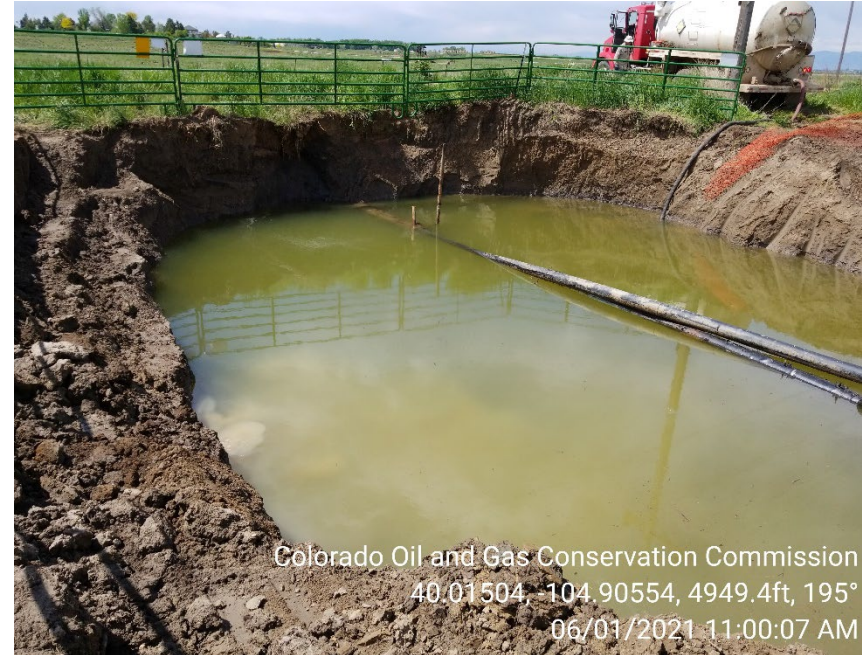
Photo 2 – Open excavation with groundwater. Impacts appear to remain in situ.
