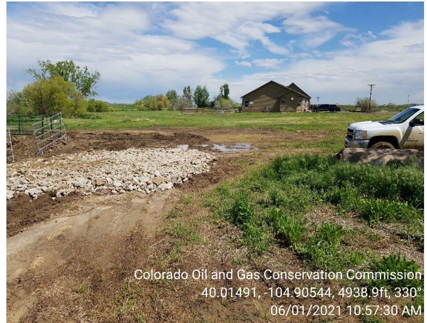
Photo 4 – Soils previously stored on location have been removed. Trash removed from location.
