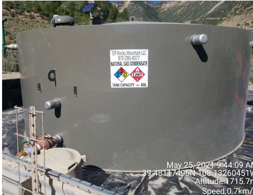
Newly installed 200 bbl Steel AST condensate tank.
