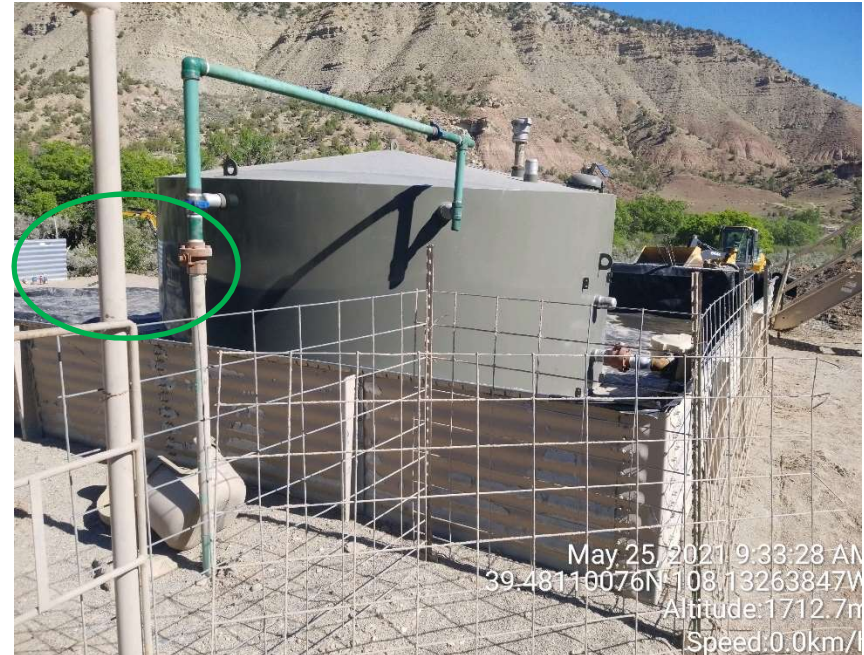
Newly installed 200 bbl Steel AST condensate tank, note the newly installed flowline that is attached to the Steel AST and the secondary containment structure in disrepair (green oval).
