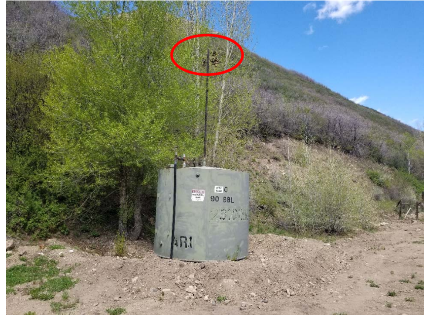
Photo 4. Venting occurring from tank labeled "vent tank."
