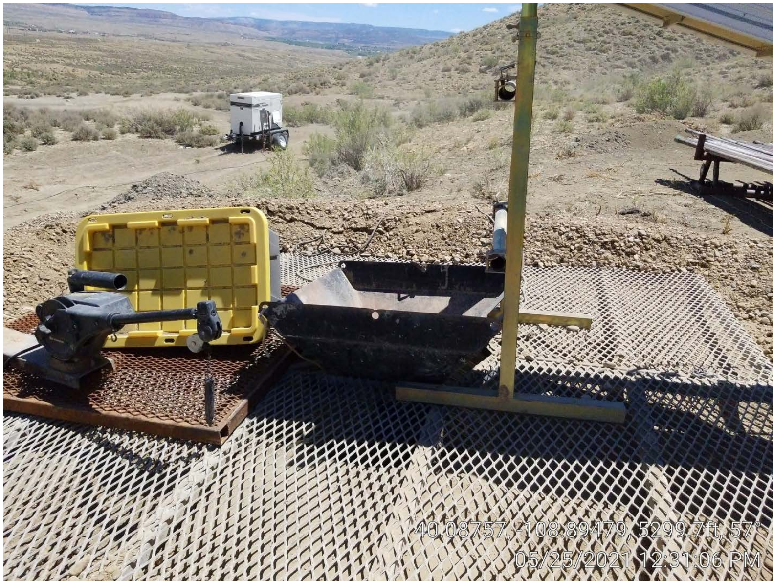
Photo 1. Gravel funneled into well.
